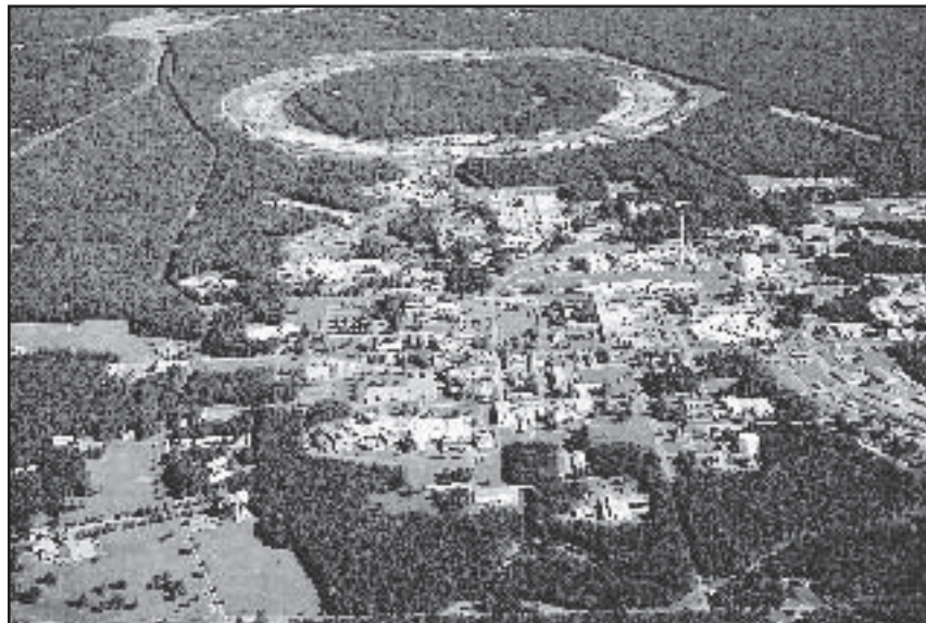
CLEAN-UP SITE: Aerial View of Brookhaven National Laboratory in the Central Pine Barrens. $41 Million will accelerate clean-up by two years.
