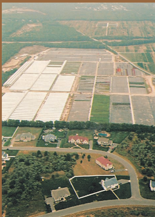
BOUGHT AND SOLD: Taxpayers thought that by purchasing the development rights, the open farm field vistas would remain. Instead, the topsoil was stripped and industrial greenhouses were erected on this “farm” in East Moriches.
